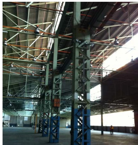
Figure 2 Photo of the original steel structure
