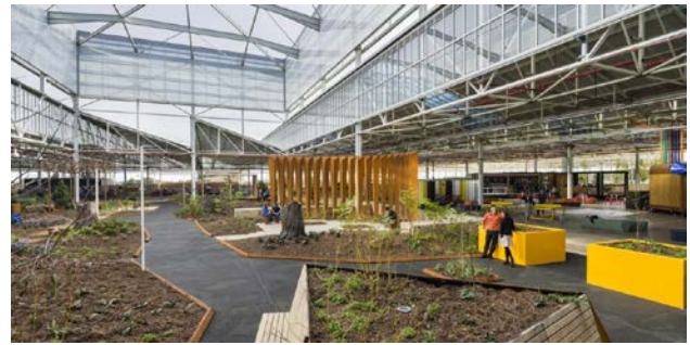
Figure 15 Completed building showing the extent of refurbishment
