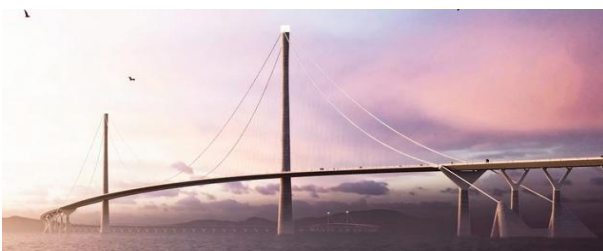
Figure 1. Lingding Channel Bridge
