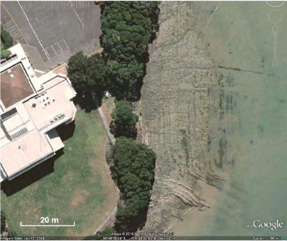
Figure 14: Google Earth aerial view from 100 m elevation showing open joint planes clearly visible in the shore platform at Chelsea sugar refinery, Birkenhead. As with the previous figure, the joint planes have opened and are vulnerable to erosion.
