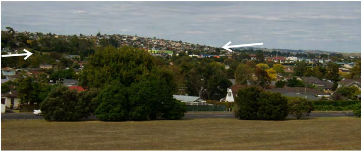
Figure 21: Approximate position of the new inferred Bucklands Beach Fault (white arrows), photographed towards the SSE from the lower slopes of Pigeon Mountain volcano. Pigeon Mountain and the houses in the foreground are situated on the downthrown Pakuranga block, west of the fault, while the slopes in the background of the photo (above the arrows) are located on the upthrown Howick block, east of the fault. The lime green building in the centre of the photo is on the fault.
